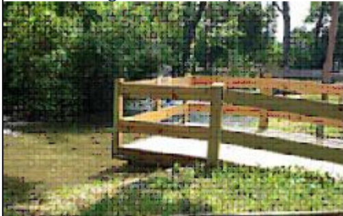
This year those fairgoers with disabilities will have access to the pond on a dock built for their enjoyment. DNR Photo by Carly Darrow
